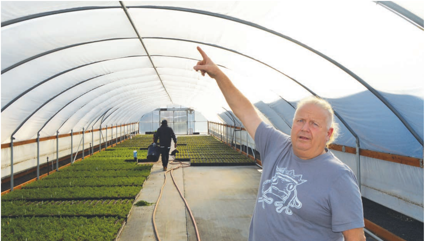
Little Prince of Oregon Nursery is phasing out Quonset style greenhouses. According to Mark Leichty (right), they add braces to every third bow in fall and winter to prevent roof collapse due to snow or ice. PHOTO BY MITCH LIES
