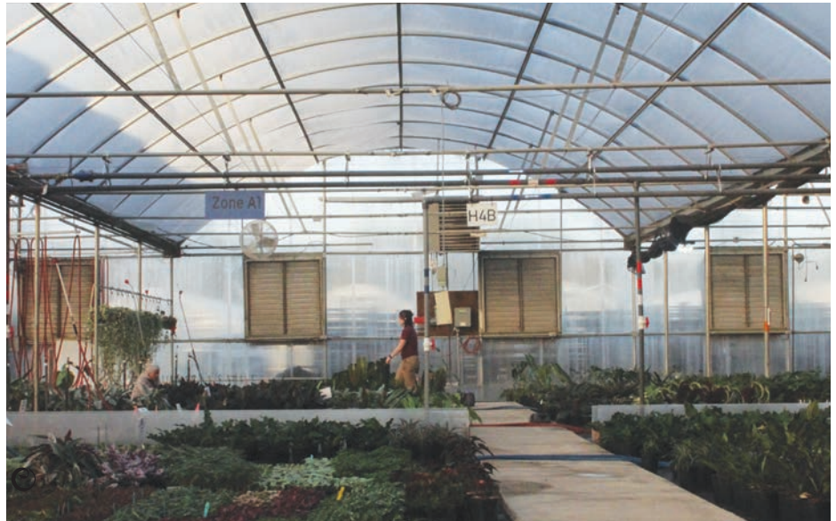
In a gutter-connected greenhouse, your sight is not limited by side walls. And because they are gutter connected, less heat is lost, Mark Leichty said. PHOTO BY VIC PANICHKUL
