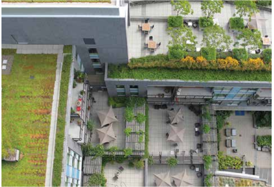
Rooftop gardens and green roofs improve air quality by trapping pollutants and reducing air temperature. PHOTO COURTESY CITY OF PORTLAND
