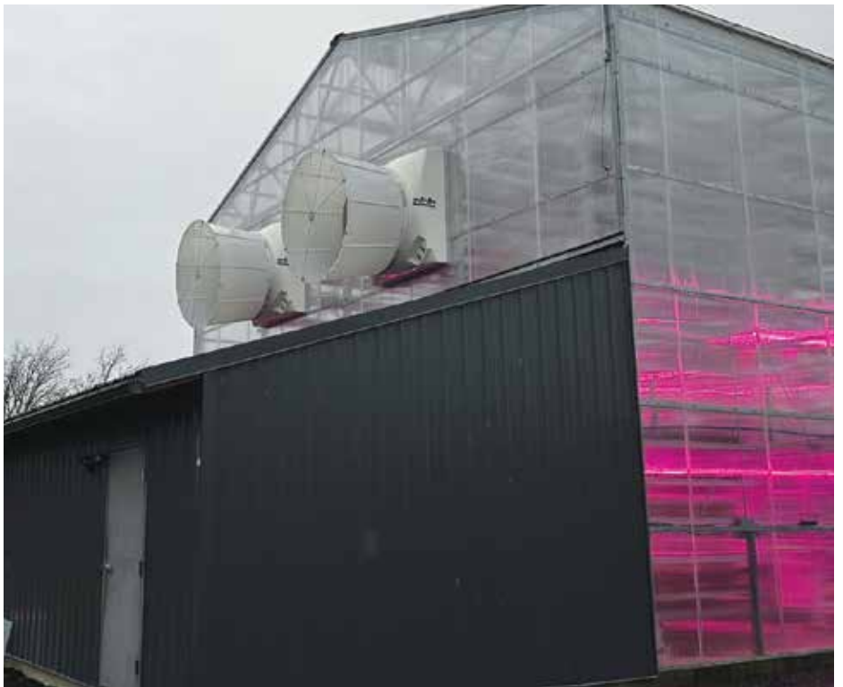
Greenhouse manufacturers like GK Machine can help calculate the ventilation and circulation systems needed for any particular greenhouse and recommend solutions. In a test greenhouse at GK's property in Donald, Oregon, small fans (above) maintain air movement within the greenhouse and larger fans (below) ventilate the greenhouse. PHOTO BY VIC PANICHKUL
