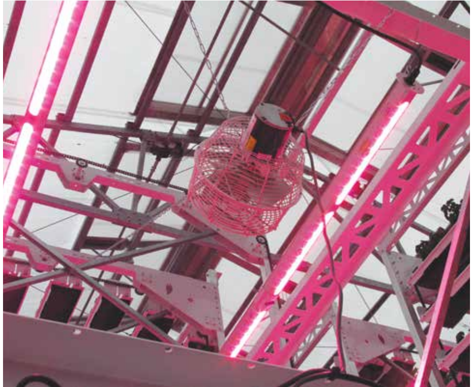
Greenhouse manufacturers like GK Machine can help calculate the ventilation and circulation systems needed for any particular greenhouse and recommend solutions. In a test greenhouse at GK's property in Donald, Oregon, small fans (above) maintain air movement within the greenhouse and larger fans (below) ventilate the greenhouse. PHOTO BY VIC PANICHKUL
