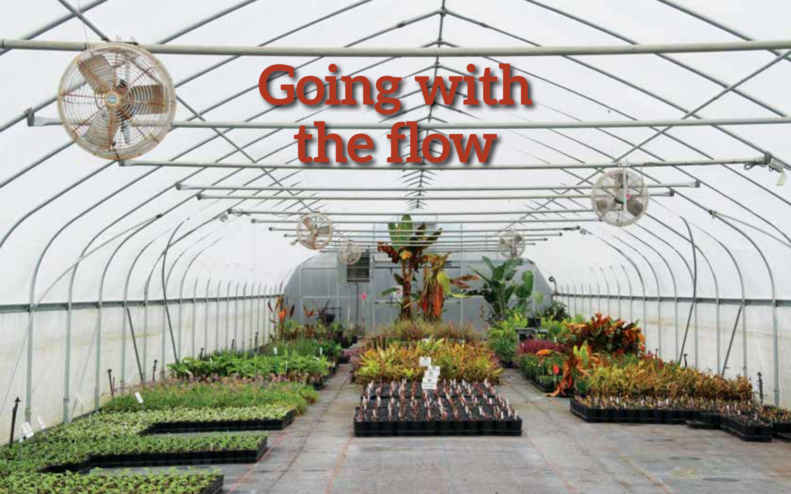
Little Prince of Oregon uses rows of small fans in each greenhouse to maintain horizontal air flow. PHOTO BY VIC PANICHKUL
