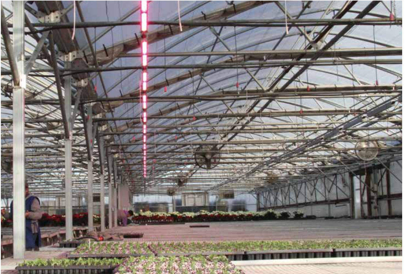
Al's Garden & Home installed LED lights at its nursery in Hubbard, Oregon, to cut back on grow time for its rooted liners and early spring crops. The nursery had previously had no artificial lighting. PHOTO BY VIC PANICKUL
